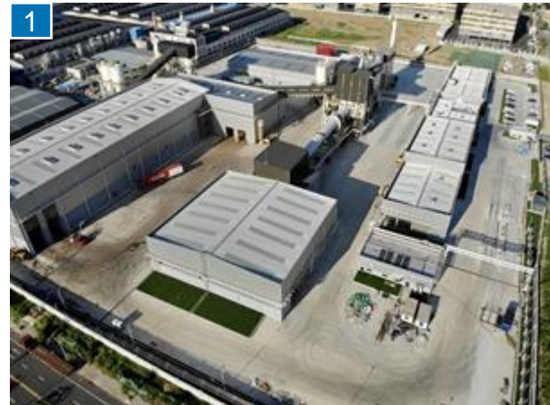
↑ Changzhou plant, completed
